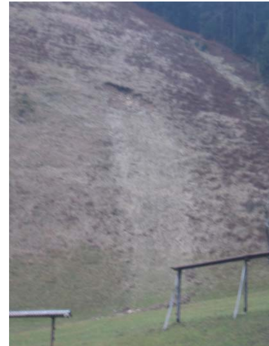
Shallow slope failures and landslides
